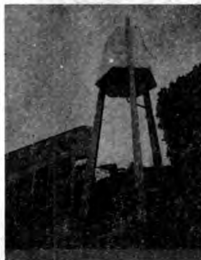
FIG 9, Overhead Water Tank
