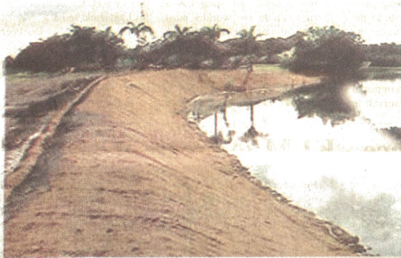
After the installation
