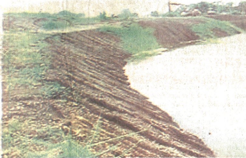
Before the installation
