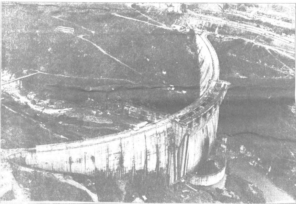
Victoria project under construction
