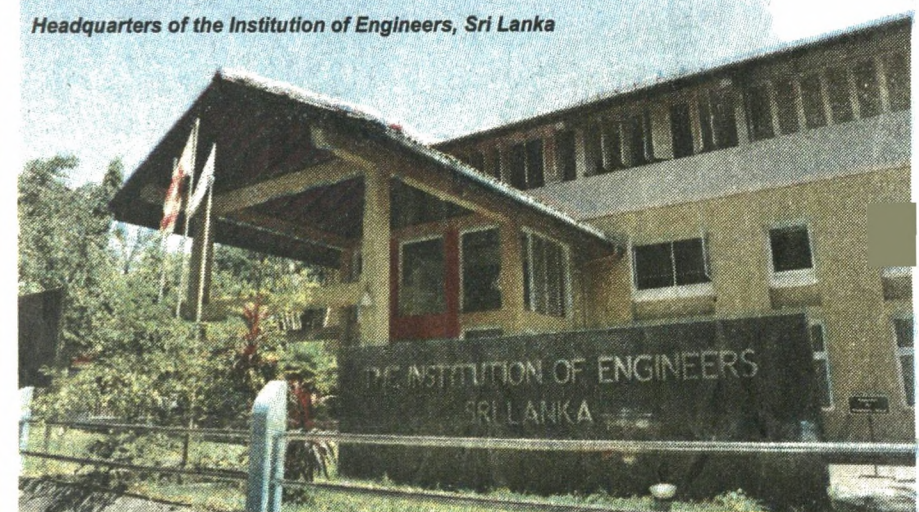
Headquarters of the Institution of Engineers, Sri Lanka
