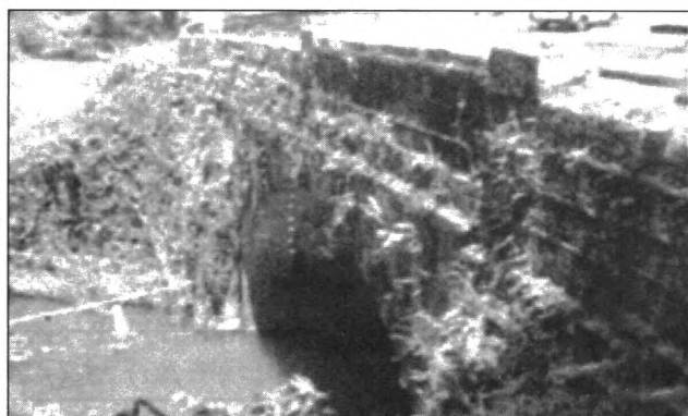
Figure 5: A view of the selected arch bridge at 71/1 along A7 road
