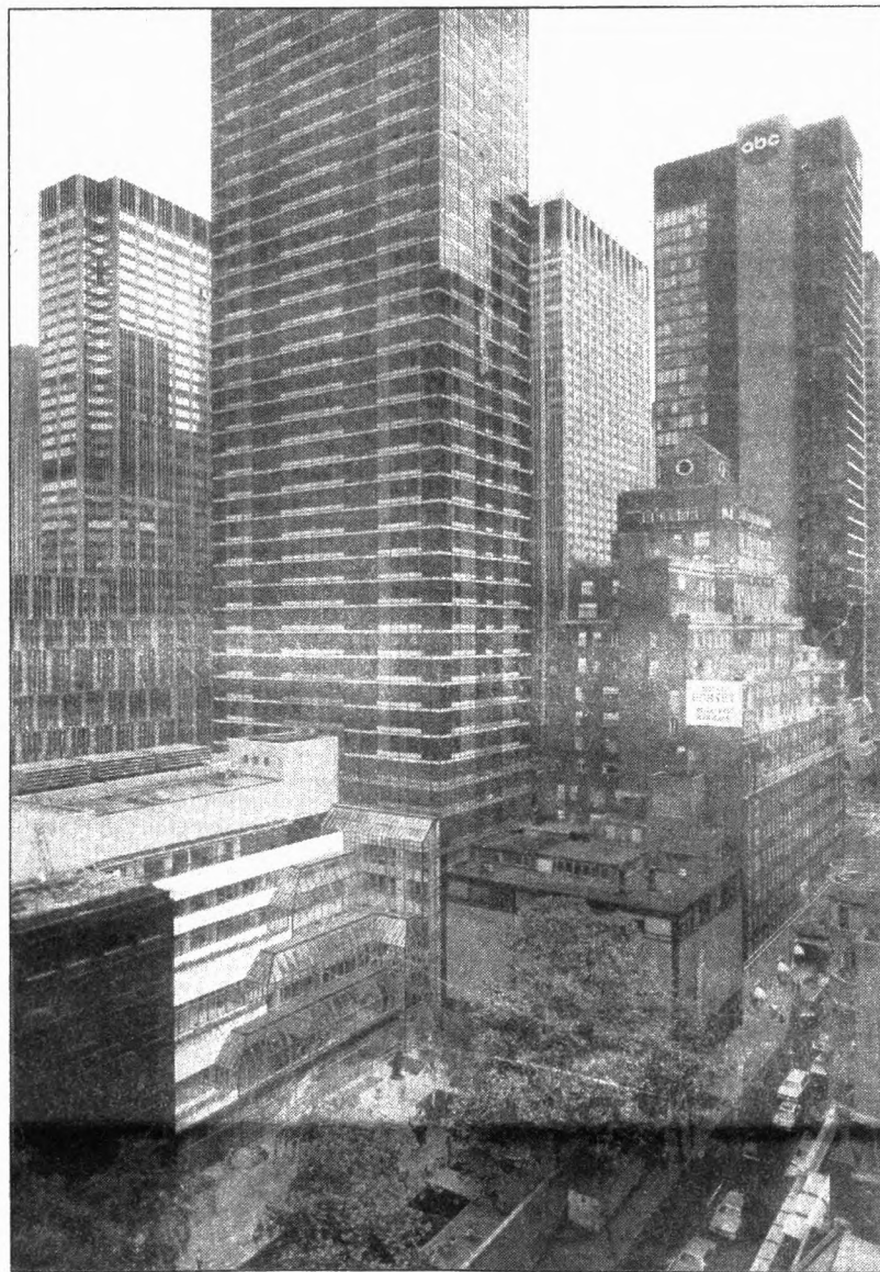
High rise buildings - looming dangers
