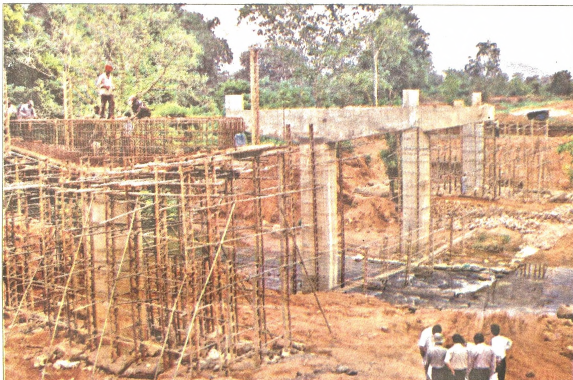
The Moragahakanda-Kalu Ganga scheme is one of the largest construction projects under the Mahaweli Development Program.
