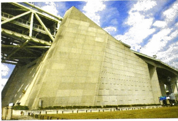
Figure 1 - Anchorage block of Akashi Kaikyo bridge.
