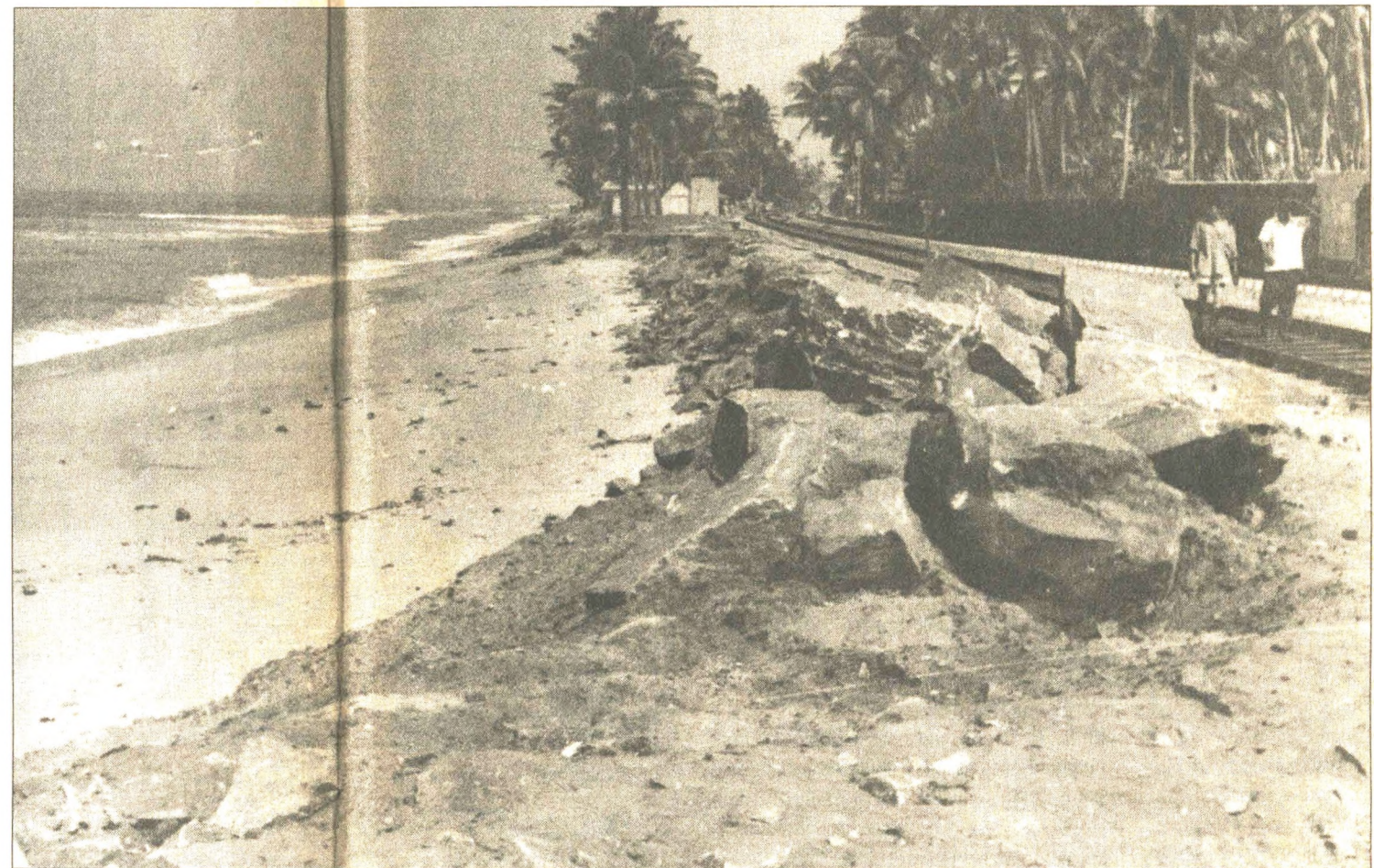
Sea erosion — mainly caused by coral mining
