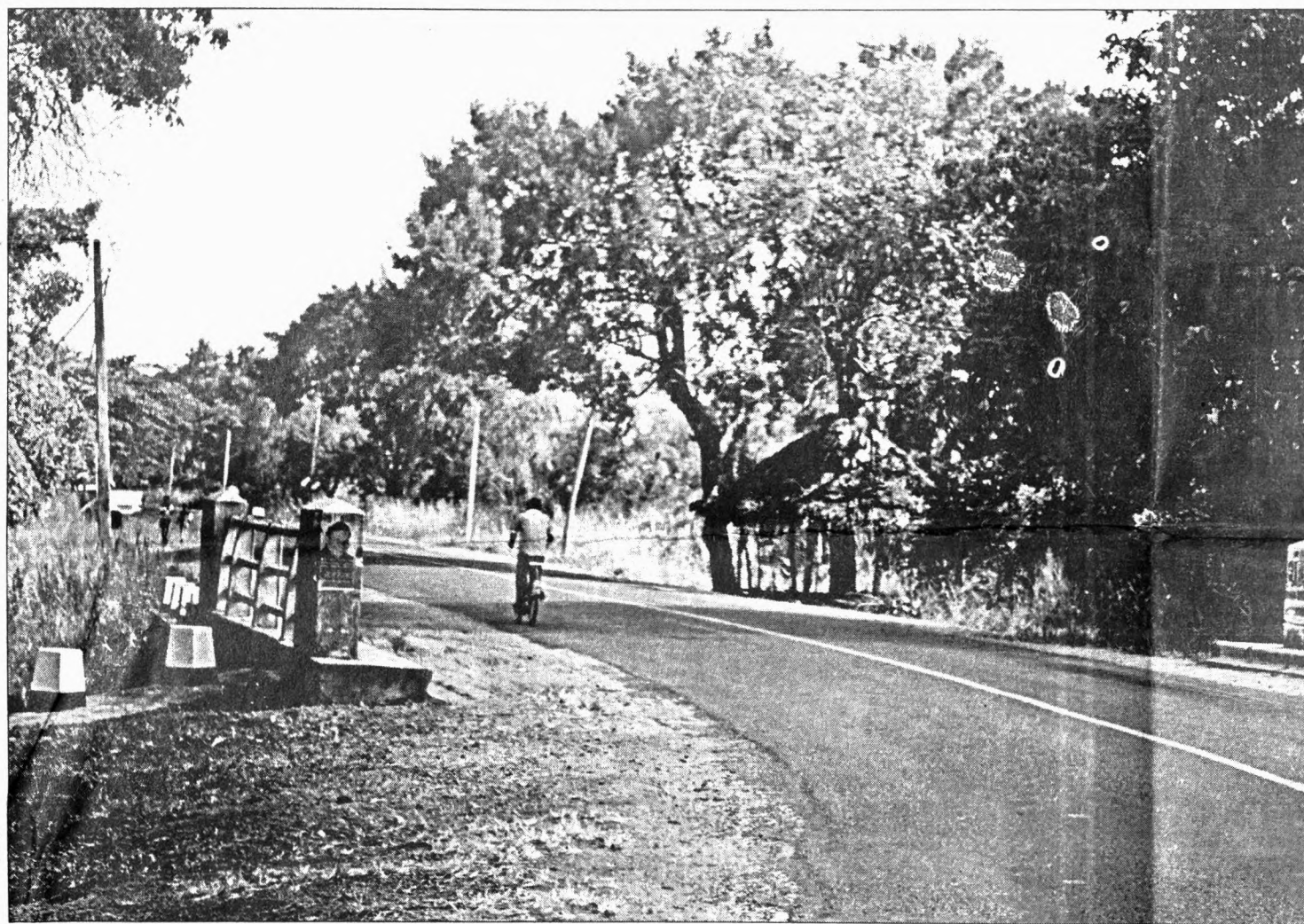
Palavi-Kalpitiya road constructed under the Maga Neguma development drive
