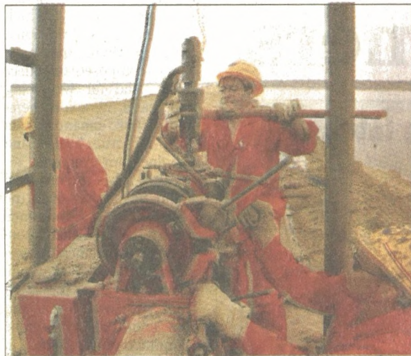
Chinese construction workers at the construction site of the new Hambantota harbor in Hambantota.
