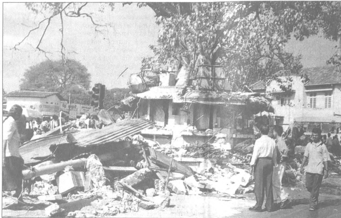
The temple at Punchi Borella being demolished by the UDA
