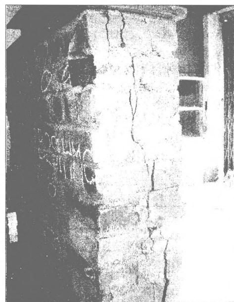
Figure 10: Tested brick panel
