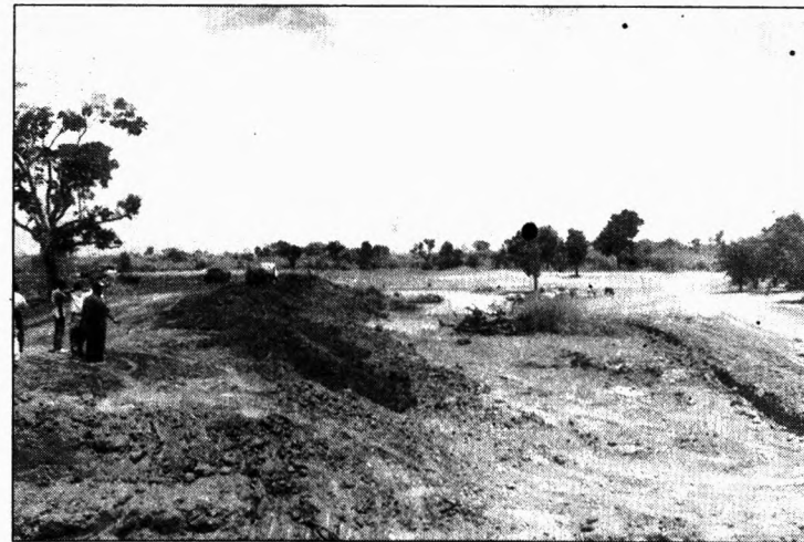
The construction work of the Gal Amuna irrigation project at Kataragama commenced recently. Irrigation and Water Management Minister Gamini Jayawickrema Perera inspected the construction work.
