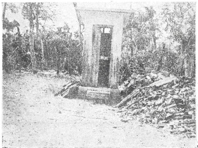
Fig. 3. External toilet (undamaged)
