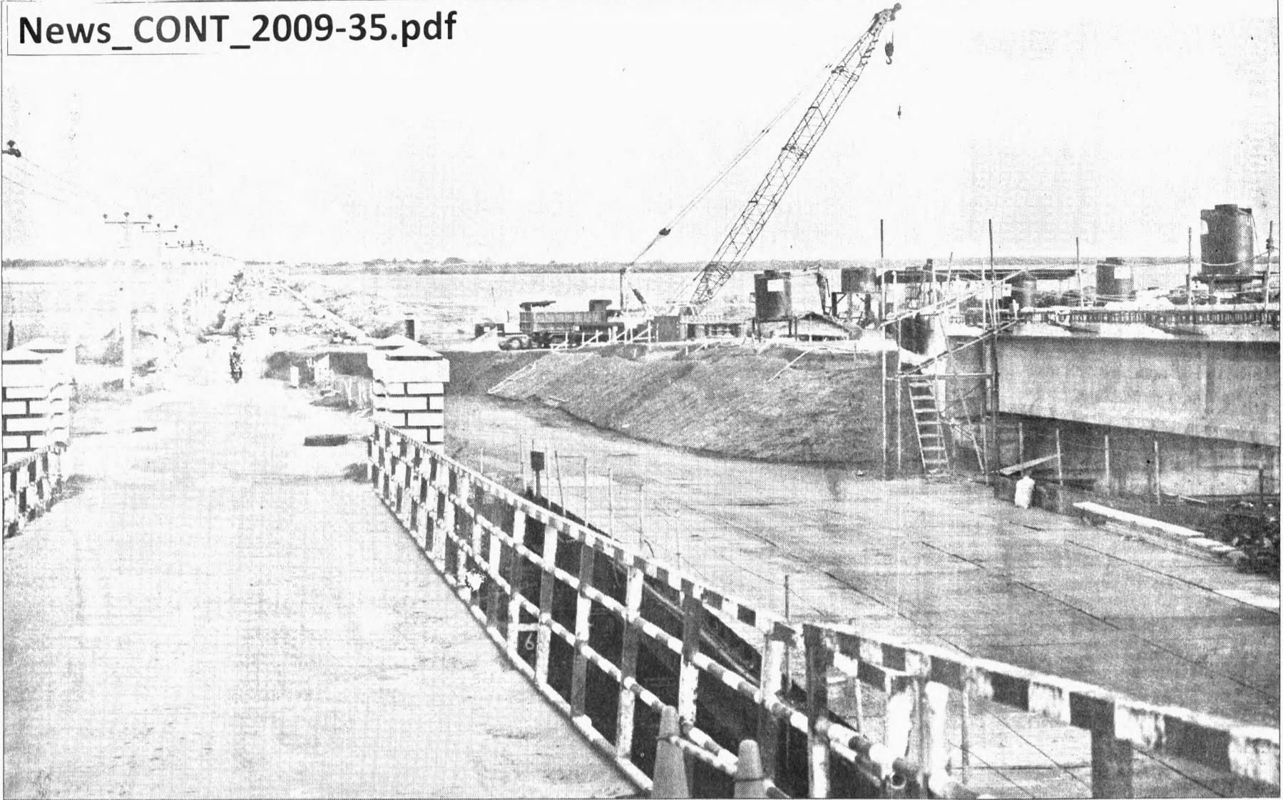
Highways and roads under construction in the North. ANCL File Photo
