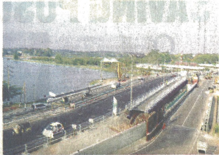
CONSTRUCTION WORK AT POLDUWA BRIDGE
