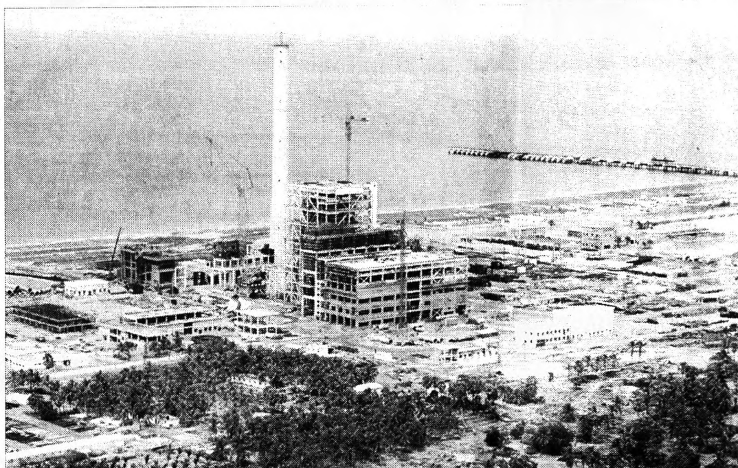
Norochcholai power plant
