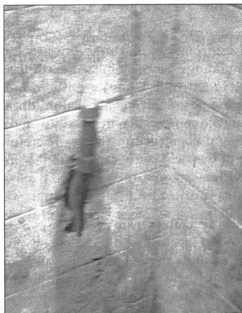
Figure 9: The problems with water lines
