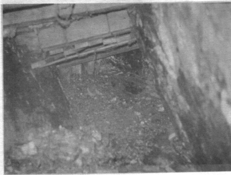
FIGURE 9 Stope roof support
