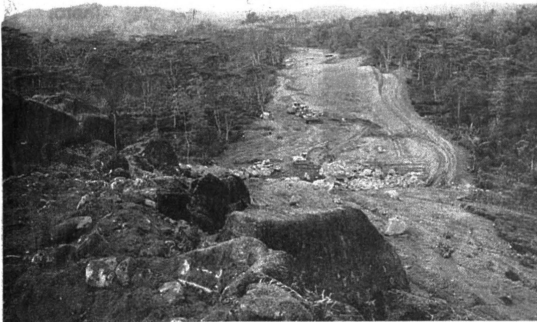
Southern Highway under construction
