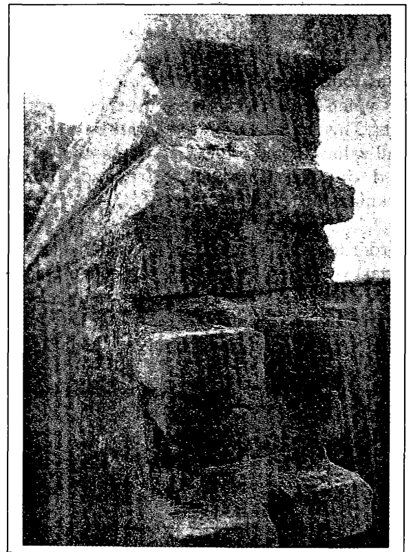
Figure 2 - A chaotic or non-standard brick wall with 'chapparau' (mortar on vertical surface of wall making it flat as a plate)
