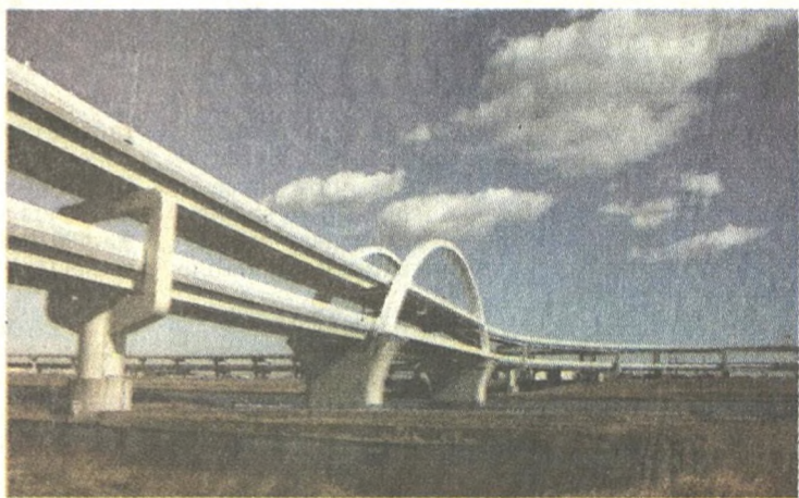
ANURADHAPURA METRO RAIL
