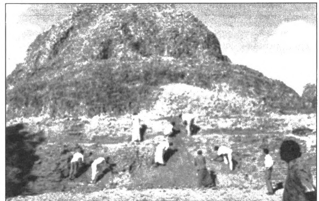
Mirisavetiya - All ancient brickworks carefully removed
