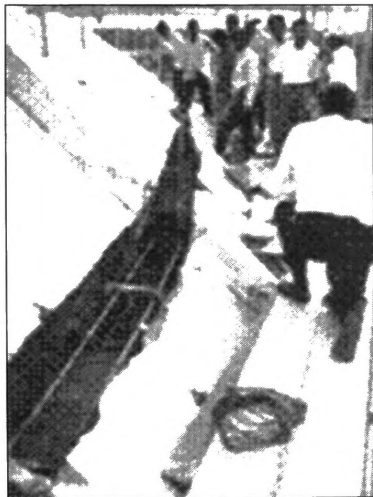
One of the Reinforced concrete rings tying up the dome under construction being inspected by Prod. Crochet
