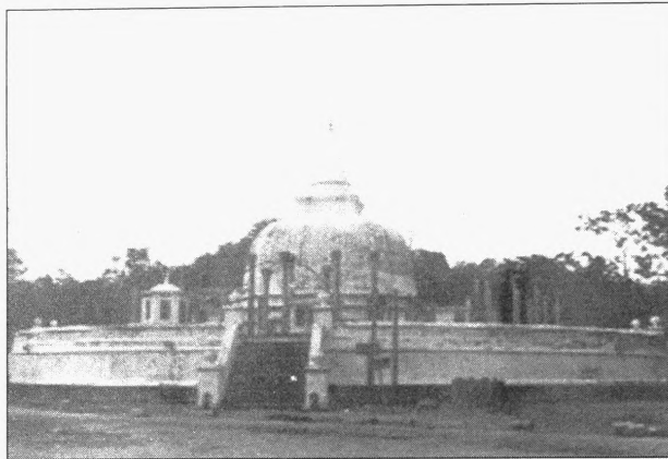
Lankaramaya - After restoration
