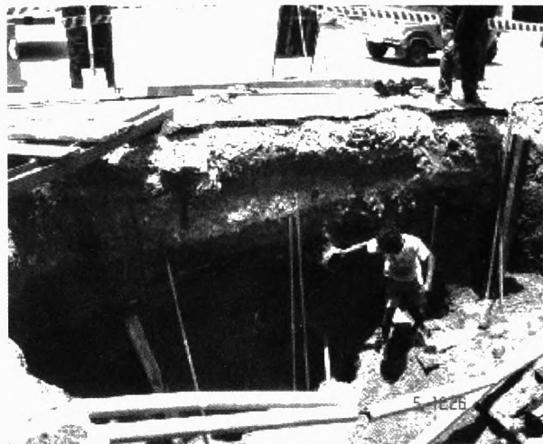
Figure 2 & 3 - Recent sewer collapse at Wellawatte
