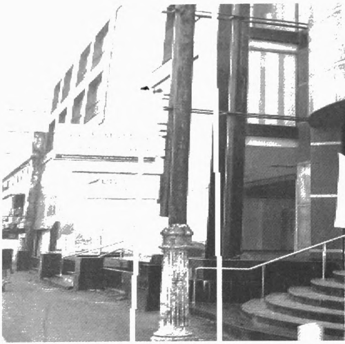
Figure 6 -Typical Vent shaft at Duplication Road
