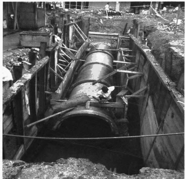
Figure 4 - Laying of Sewer Pipe Lines on a graded fill
