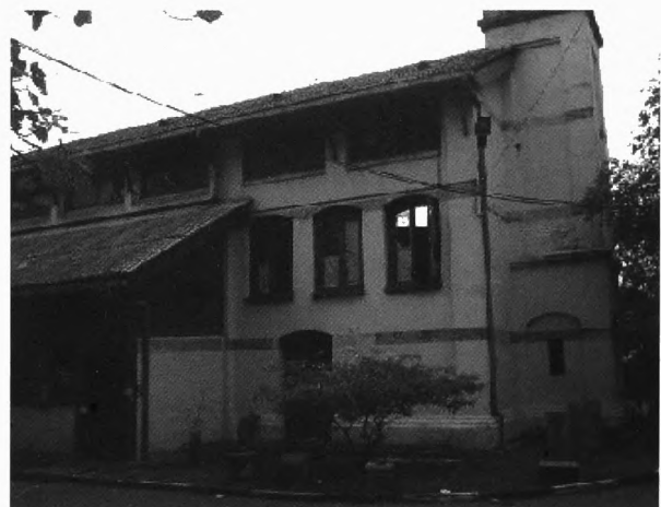
Figure 7 - One of the pumping station in Colombo
