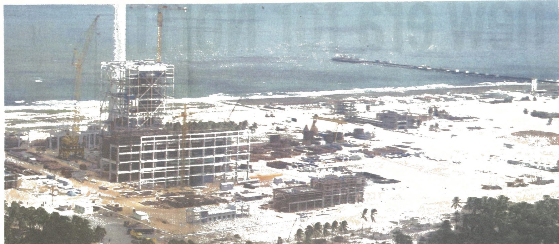
Construction of Sri Lanka's first coal power plant in Norochcholai in progress.
