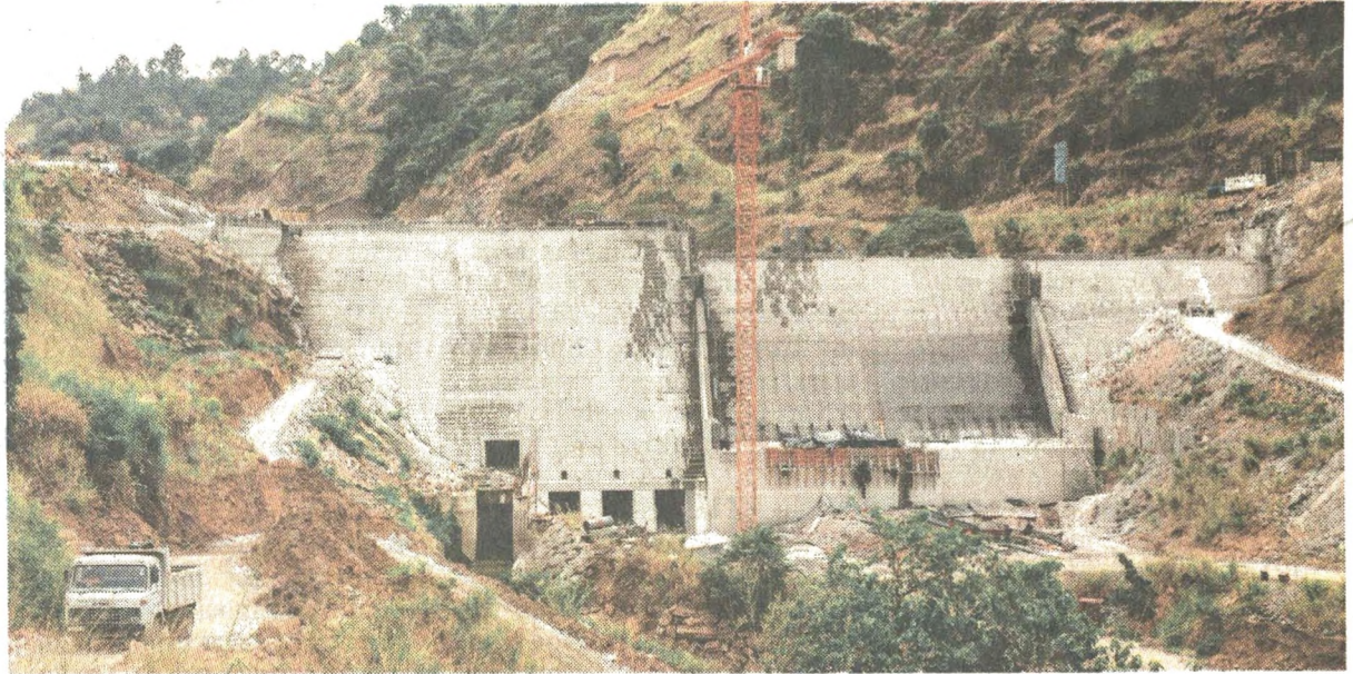
The Dyraaba dam, which is now over 80 per cent complete.
