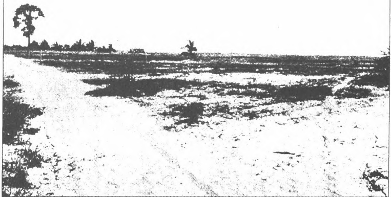
File photo: Proposed site for Norochcholai power plant. Putting up a power plant in Kalpitiya area is like sitting an important project on the top of a not-so-dormant volcano.
