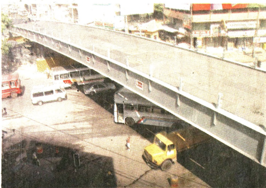
The Nugegoda flyover will be opened on January 22 to overcome traffic congestion in the area. The Road Development Authority coordinated the construction and it was built by Access Engineering. The flyover, the second after Kelaniya, consists of two lanes. Construction work commenced on October 10 with an investment of Rs. 840 million.
